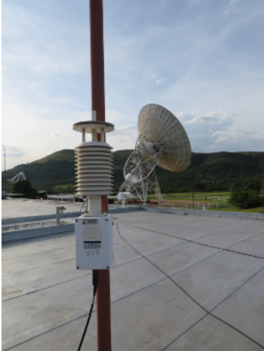
Fig. 2 The Paroscientific MET3 unit of the HRAO IGS GNSS station used in the comparison is located on the roof of the main building. The new MET4 is temporarily installed \sim 12 m behind the MET3, in the direction of the 26-m antenna in the background.
