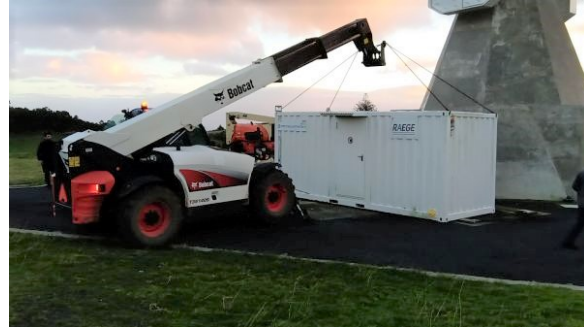
Fig. 5 Replacement of RAEGE Santa Maria radiotelescope servo container.
