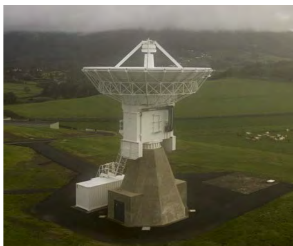
Fig. 4: Santa Maria 13.2 m station from a drone.
