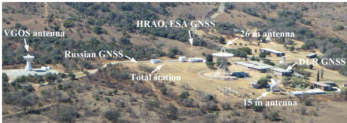
Fig. 2: VLBI local tie observing system – components of measurement and reference networks.
