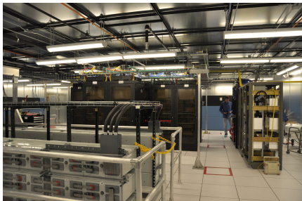
Left: WIDAR during construction
